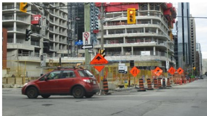
Construction all around the War Museum
